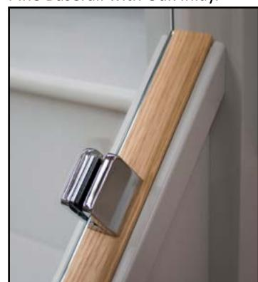
Baserail Infill and Glass Clamp detail.
